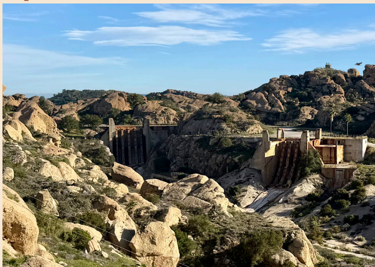
The former Coca IV (left) and Coca I (right) test stands following completion of Phase 6 and Phase 7 demolition. Remaining concrete pads, foundations, and asphalt are planned for removal as part of Phase 8.
