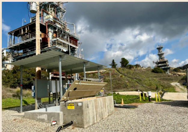
Pictured above: NASA's enhanced in situ bioremediation (EISB) system, which relies on naturally occurring microbes to remove TCE. EISB is one of the multiple treatment methods proposed in the Phase 1 CMS.
