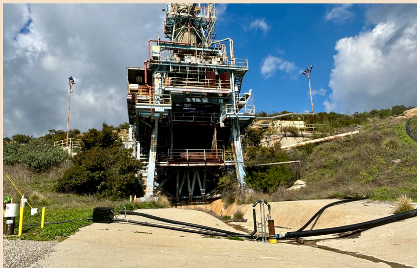
The EISB pilot system relies on naturally occurring microbes to remove TCE and other VOCs from the groundwater beneath the Alfa Test Area in NASA's Area II at SSFL.
