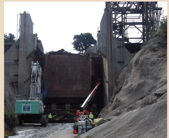
Demolition crews are shown taking apart, piece by piece, the metal flame bucket located at the bottom of Test Stand 4.
