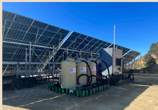
Vapors are pulled through the bedrock and pumped from the extraction well into these containers of activated carbon where they are treated.
