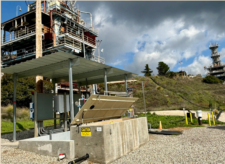
Enhanced in situ bioremediation (EISB) is one of the remedies selected in NASA's Phase 1 Groundwater CMS. NASA built a pilot EISB system (pictured above) near the spillway of Alfa 1.
