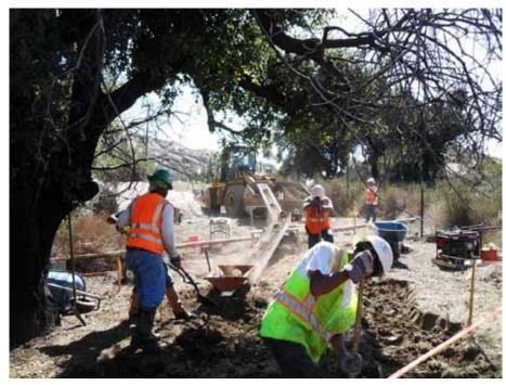
Soils were removed from the excavation area by wheelbarrow and conveyor belt Soils were loosened with hand tools
