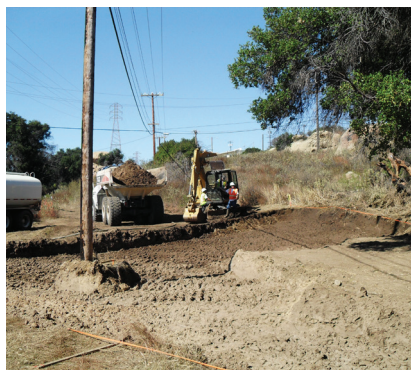
This photo from a 2012 NASA Interim Soil Removal Action illustrates the need for clean soil backfill for the restoration and revegetation of the native habitat in areas requiring soil removal.
