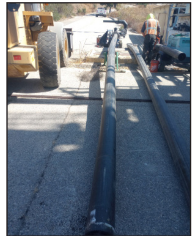
Workers prepare the high-density polyethylene pipeline (HDPE) for the Bedrock Vapor Extraction pilot study system in the Alfa Test Area.
